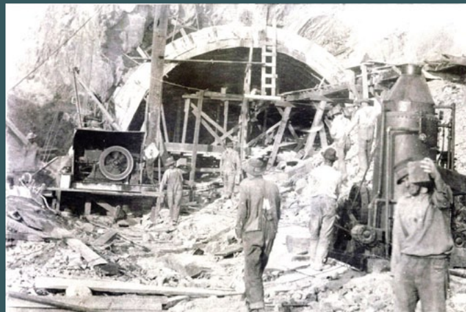
Building the Ferry Point Tunnel in 1914
