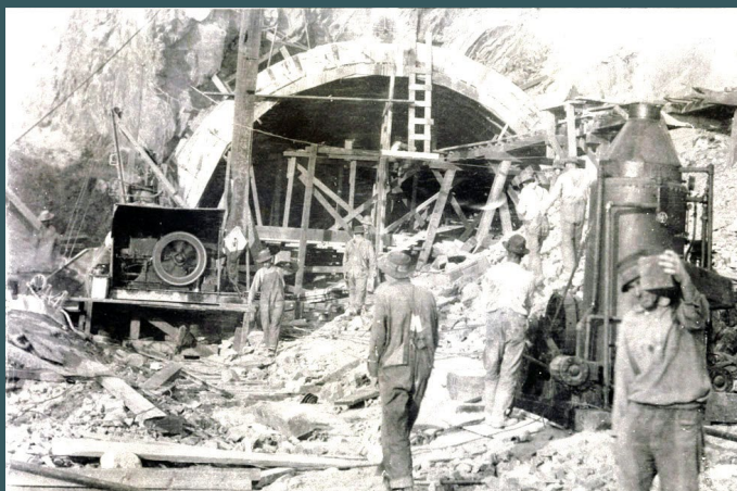
Building the Ferry Point Tunnel in 1914
